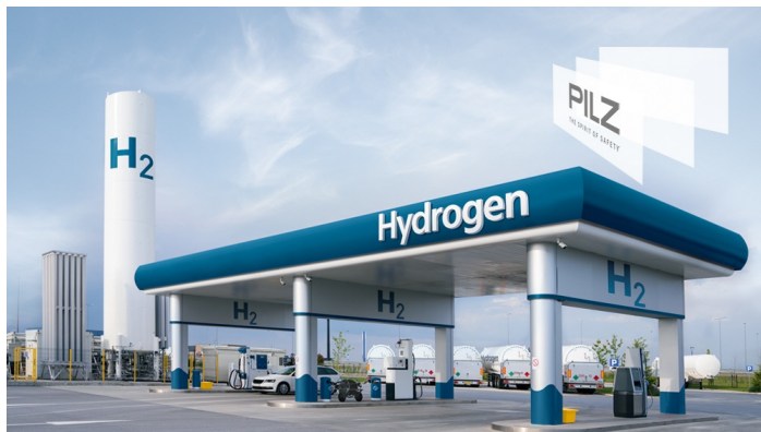
Caption: Safety solutions from Pilz are used to detect hydrogen leaks, flames and smoke, and to monitor temperature and pressure on hydrogen refuelling stations. (Photo: © iStock.com/Scharfsinn86, Pilz GmbH & Co. KG)
